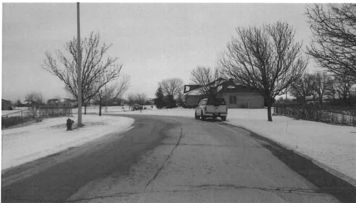
Photo # 2 - Looking east toward bridge
