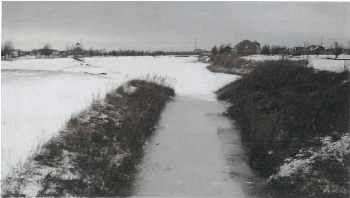
Photo # 4 - Looking upstream from bridge
