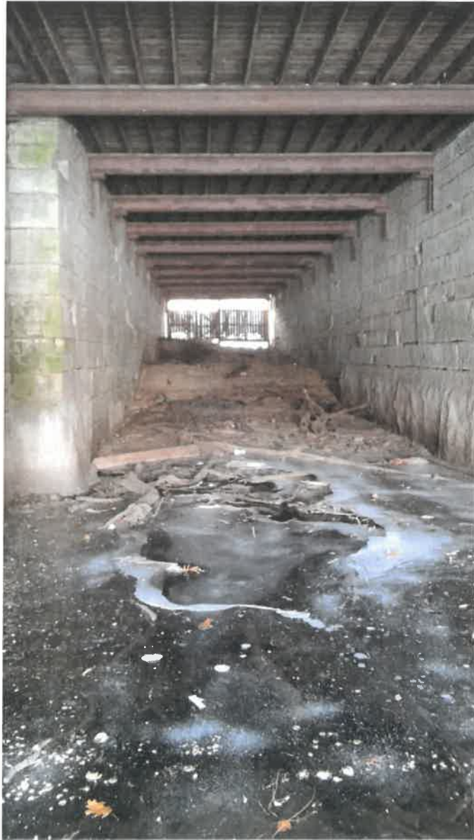
Photo # 15 - Looking south under east span
