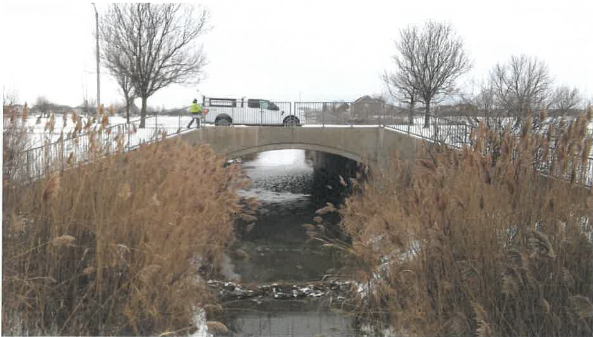
Photo # 8 - Looking upstream toward bridge
