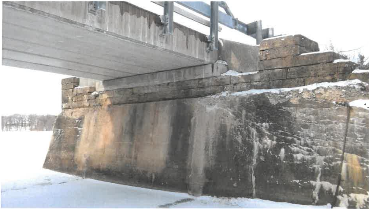
Photo # 1 - Facing southwest toward west abutment
