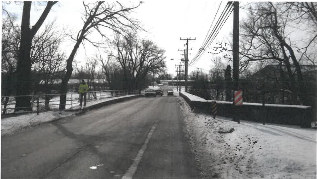
Photo # 4 - Looking south toward bridge
