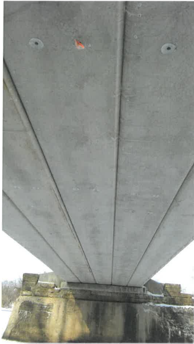
Photo # 6 - Looking west beneath west span
