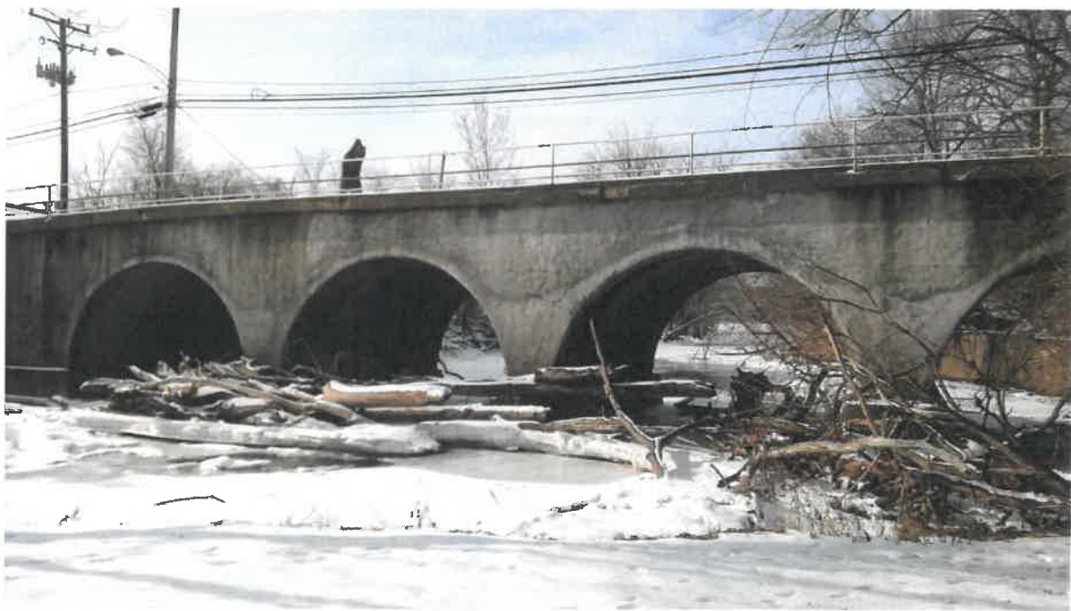
Photo # 5 - Looking downstream toward bridge
