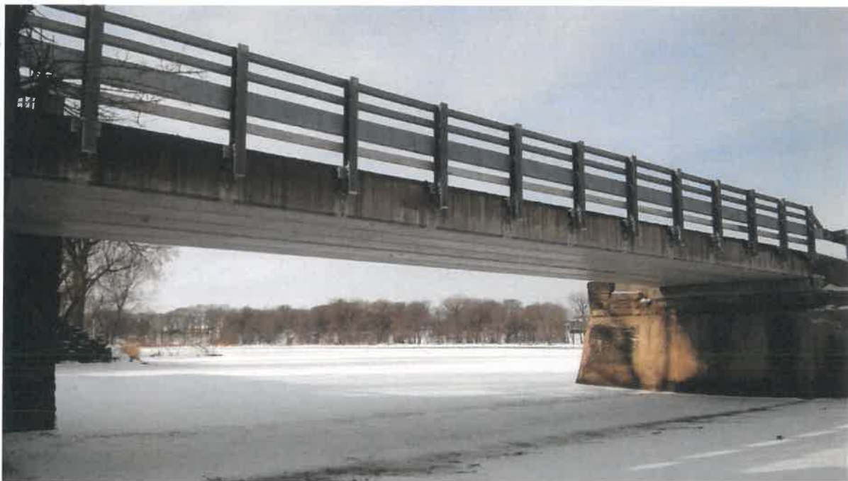
Photo # 8 - Looking south toward west span
