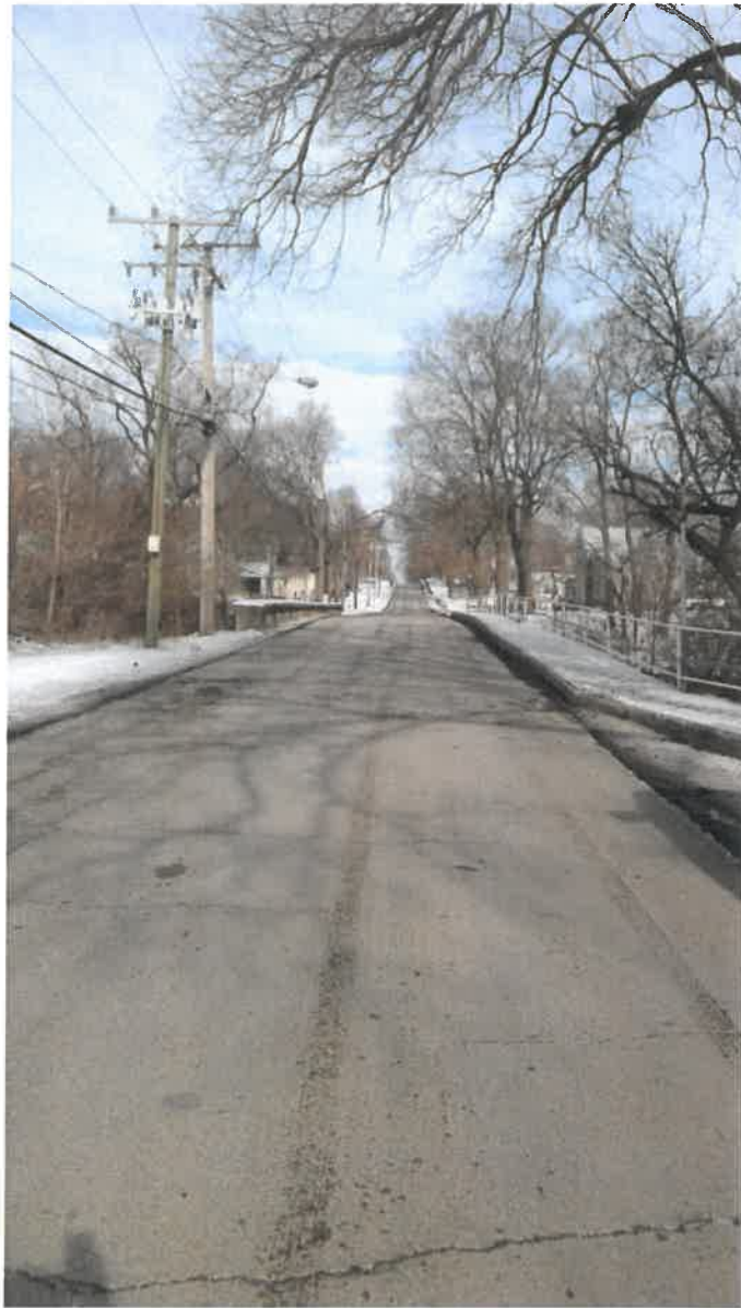
Photo # 1 - Facing north toward bridge
