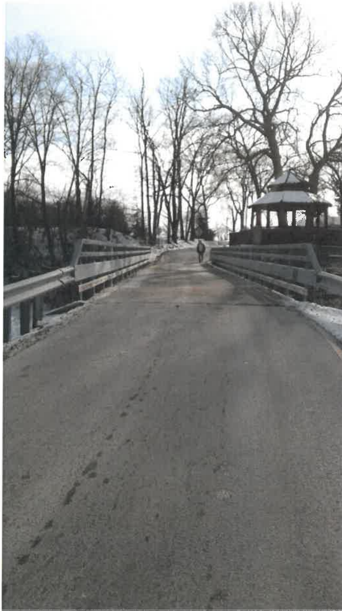
Photo # 14 - Looking east toward bridge
