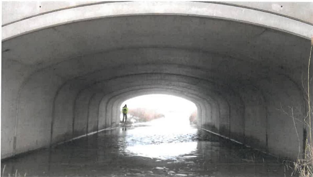
Photo # 6 - Looking upstream thru bridge
