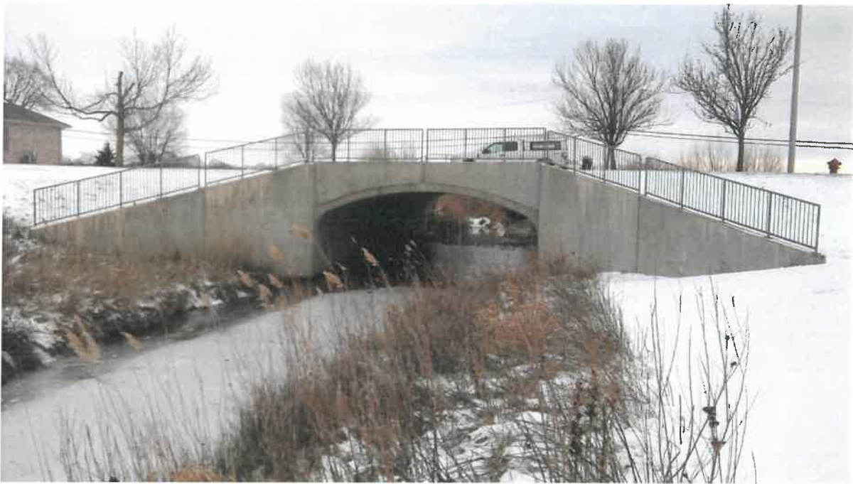
Photo # 7 - Looking downstream toward bridge
