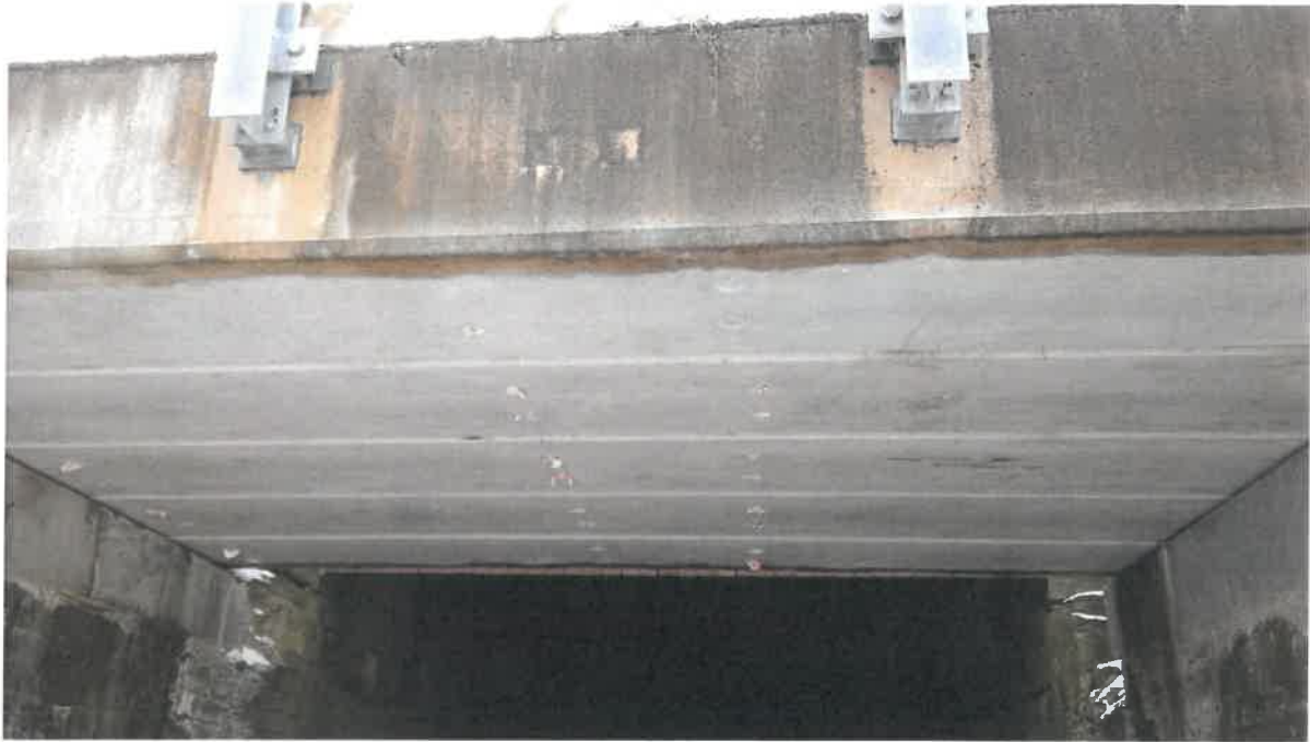
Photo # 7 - Looking south toward east span
