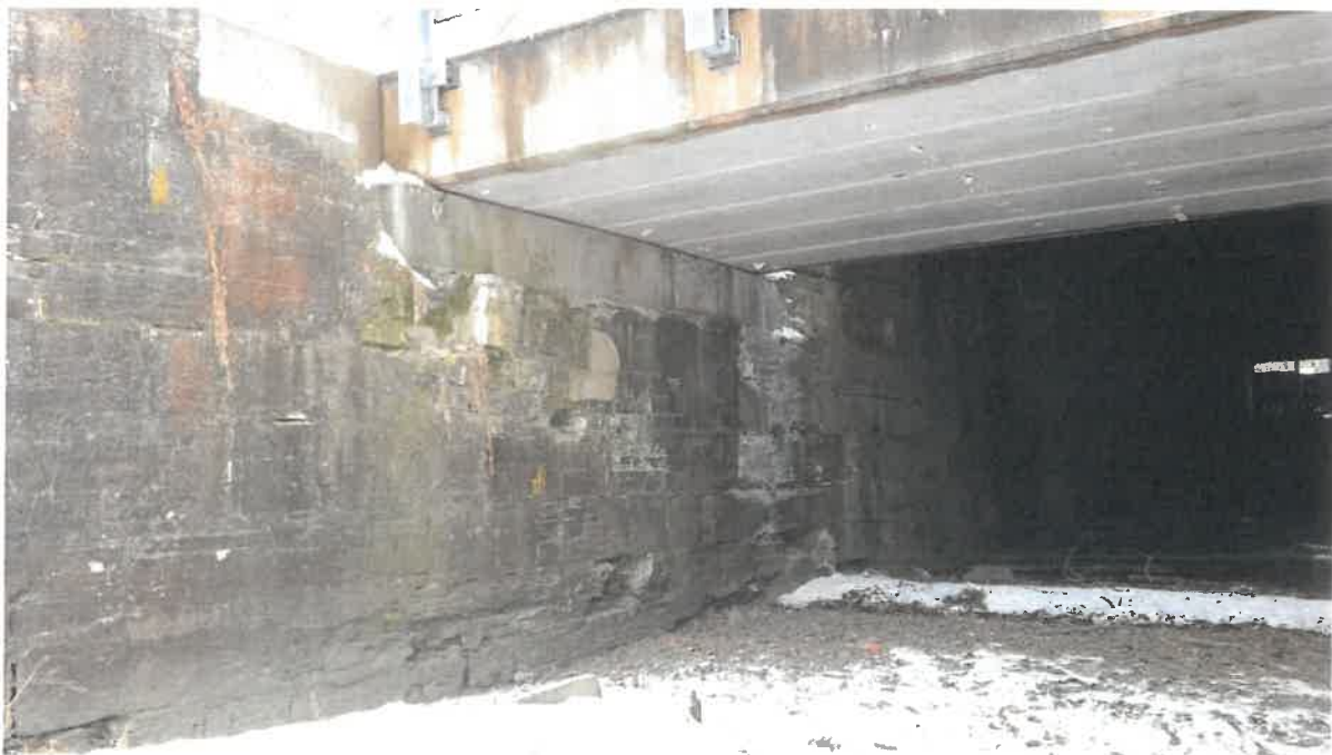
Photo # 5 - Looking southeast toward east abutment
