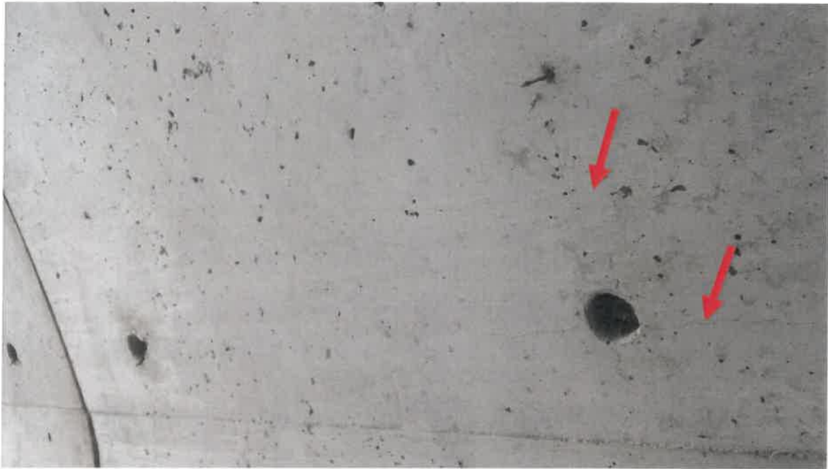
Photo # 5 - Hairline cracks at east end of 2nd arch from upstream end
