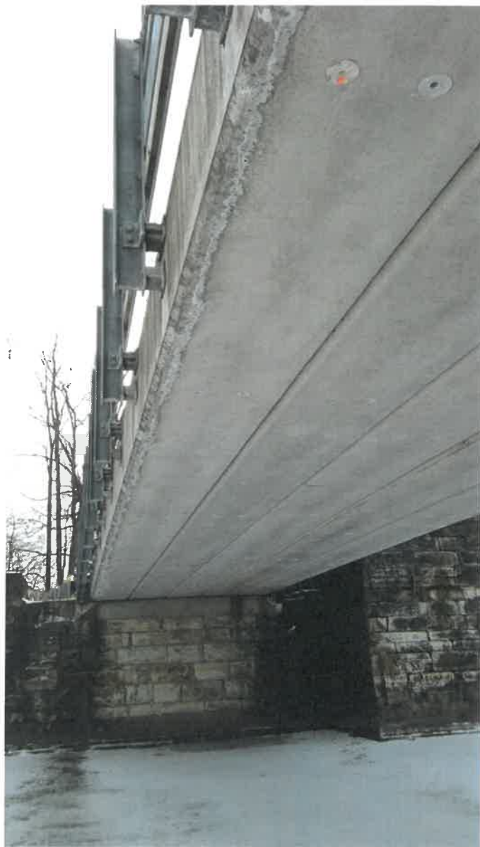
Photo # 3 - Facing east beneath west span
