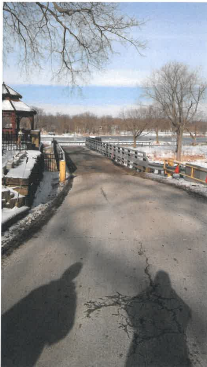
Photo # 12 - Looking west toward bridge
