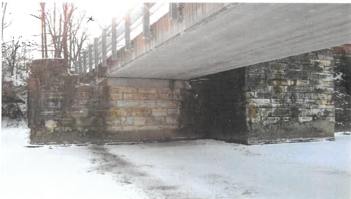
Photo # 2 - Facing east toward pier
