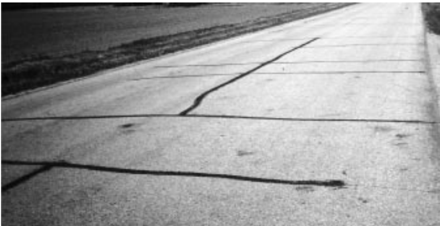
▼ Open crack, 1/2" wide; adjoining pavement sound.
